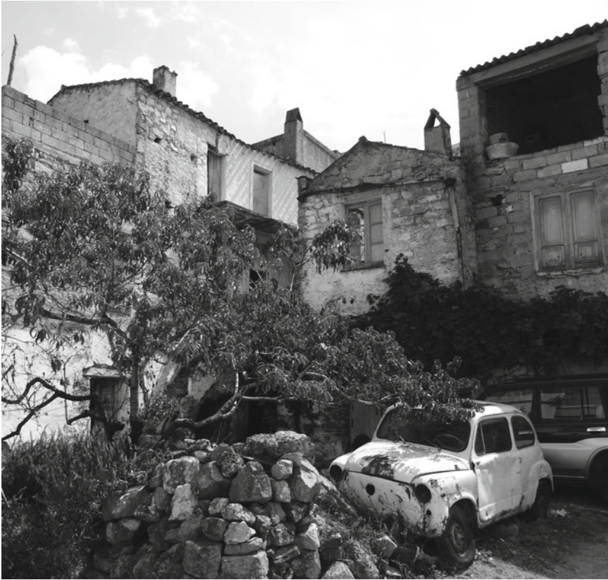
Fig. 1 The number of condemned building is progressively increasing ( source photo by the Authors)
