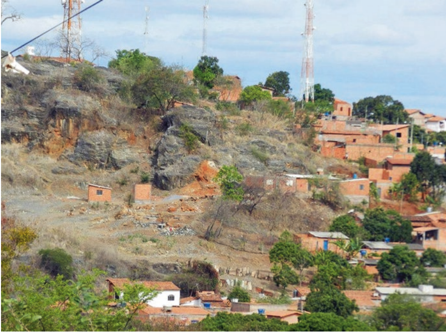
Fig. 5.19 Recent constructions in the hills near Montes Claros in 2015. (Reproduced with permission from Bolay)
