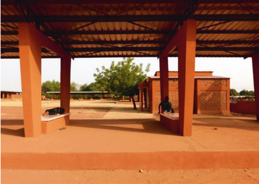
Fig. 2.15 The new bus station, Koudougou, Burkina Faso 2014. (Reproduced with permission from Bolay)
