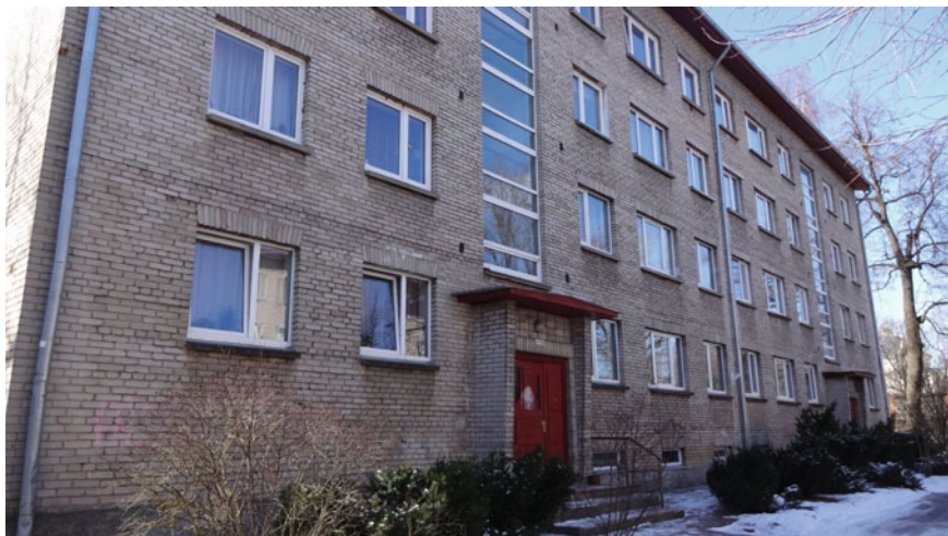
Fig. 17.1 A khrushchëvka apartment building in Tartu, Estonia prior to renovation (Tiigi 7, Tartu): a 4-storey, 32-unit building with 1,350 m 2 total floor space (an estimated 80 inhabitants live in the building). Source Photo by authors
