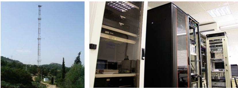
Fig. 2. (left) High (70 m) mast within the campus of NCSR D, hosting the macro-cell base station; (right) Cloud/SDN infrastructure in NCSR D
