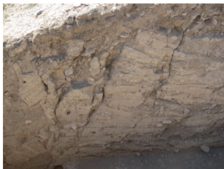
Fig. 7.6 Rammed earth wall of Tossor fortress (Lake Issyk Kul, Kyrgyzstan) as seen in excavation trench cross-cutting the buried wall. Layers are marked by horizontal scratches made by the excavating archaeologist. Three ruptures dissect the wall. Trench is 2.5 m deep (Photo M. Kázmér, #1246). For details see Korzhenkov et al. (2016)
