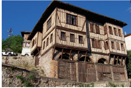
Fig. 7.11 Timber-laced masonry house in Safranbolu, Turkey ( hımış construction). The ground floor is unreinforced masonry, followed by two floors of intricate timber structure. Note oblique timbers at corners, providing support against lateral shaking. Photo Uğur Başak. Source https://commons.wikimedia.org/wiki/File:Safranbolu_traditional_house_1.jpg . Creative Commons license. Accessed September 23, 2017
