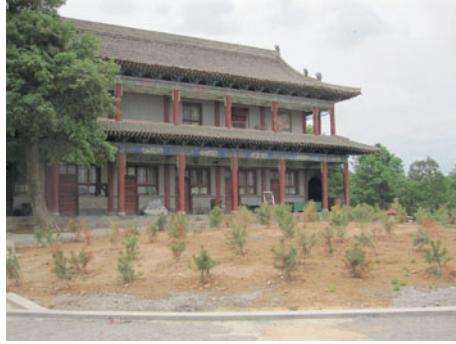
Fig. 7.9 Timber frame with masonry infill in a residential building in the Buddhist monastery at Tianshui, Gansu, China. This structure is extremely resistant to earthquakes: well-jointed columns and beams maintain structural integrity, although masonry infill might get loose under strong seismic shaking (Photo M. Kázmér, #3068)
