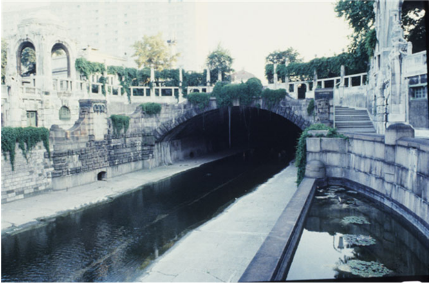
Fig. 6 At grade view of the Vienna River adjustments ( Wienflußregulierung ), including a partial view of the subterranean passage. Image courtesy of Axel Föhl; released under a Creative Commons Attribution-NonCommercial-NoDerivatives 4.0 International License
