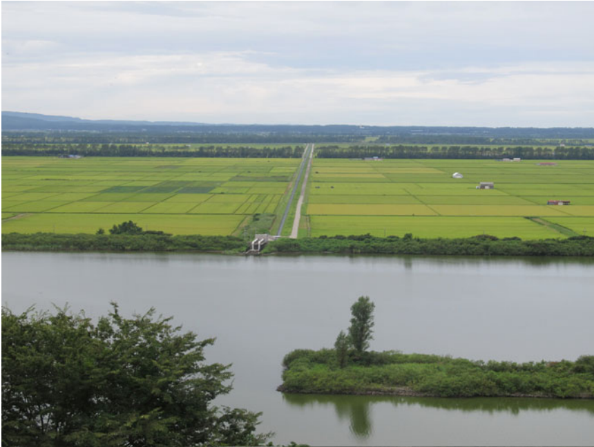
Fig. 2 Hachirogata central polder. A pump station and drainage is in the center of the photograph (Photo by Yasunori Kitao); released under a Creative Commons Attribution-NonCommercial-NoDerivatives 4.0 International License
