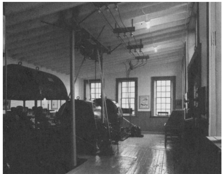
Fig. 7. The first hydroelectric development in Newfoundland was built at Petty Harbour, and electricity was transmitted to St. John's for the first time on April 19, 1900. The original equipment consisted of a Pelton wheel turbine, which was connected to a 250kVA General Electric generator. In 1907, a second Pelton wheel turbine and a generator similar in size to the original were installed. To meet increased demand and to provide for further expansion of the system, the building was extended in 1914 and a Voith turbine and a 500 kVA Westinghouse generator were installed. (Courtesy, Newfoundland Light & Power Co. Limited.)
