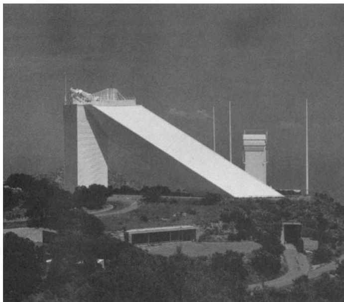
Fig. 10. Heliostat support tower and part of water-cooled wind shield of the McMath-Pierce solar telescope. (Kitt Peak National Observatory.)
