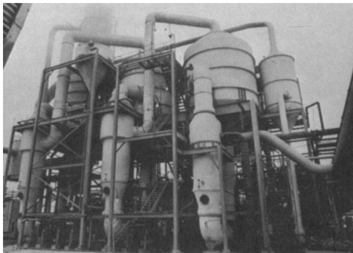
Triple-effect evaporator used in concentrating soda solutions and preparation of solid sodium hydroxide.
