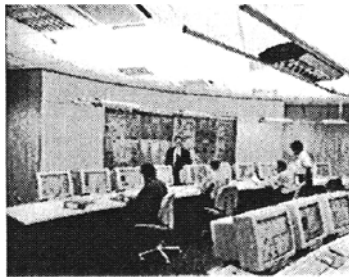
Figure 1 – Training Center for Power Plant Operator (SimPower Simulator Systems GmbH)
