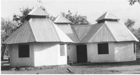
Fig. 18. Office building in Mali, based on three augmented rhombicuboctahedra and two tetrahedra, with a frame construction of palm wood
