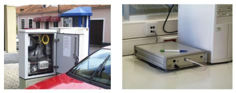
Fig. 6. BBL AS-ONU mounted on a street cabinet and a VDSL modem (NT-51).
