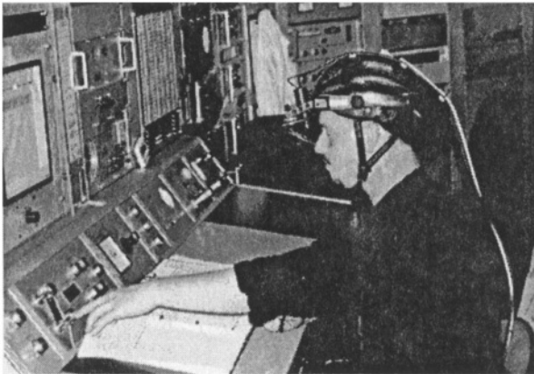
Figure 1. A nuclear control room operator wearing the eye-tracking helmet.
