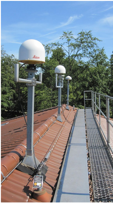
Fig. 4 Installation of GNSS antennas on the rooftop of PTB’s clock hall. The direction of view is toward the northeast. Starting from the new PTBB antenna in the foreground, we see toward the background the antennas of receivers PT09, PT10 of type MESIT GTR51 and GRCP of type MESIT GTR55, respectively
