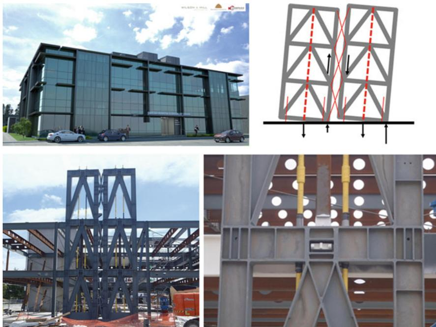
**Fig. 13.34** Forté Health Medical Centre, three storey building with over 5,000 m<sup>2</sup> of specialist medical facilities. Post-tensioned steel rocking coupled ‘walls’ (or braced-frames) in both directions, combining hysteretic and viscous dampers in parallel for “an advanced flag-shape” system. *Bottom right:* secondary interior moment-resisting frames implementing a sliding hinge joint beam-column connection solution
