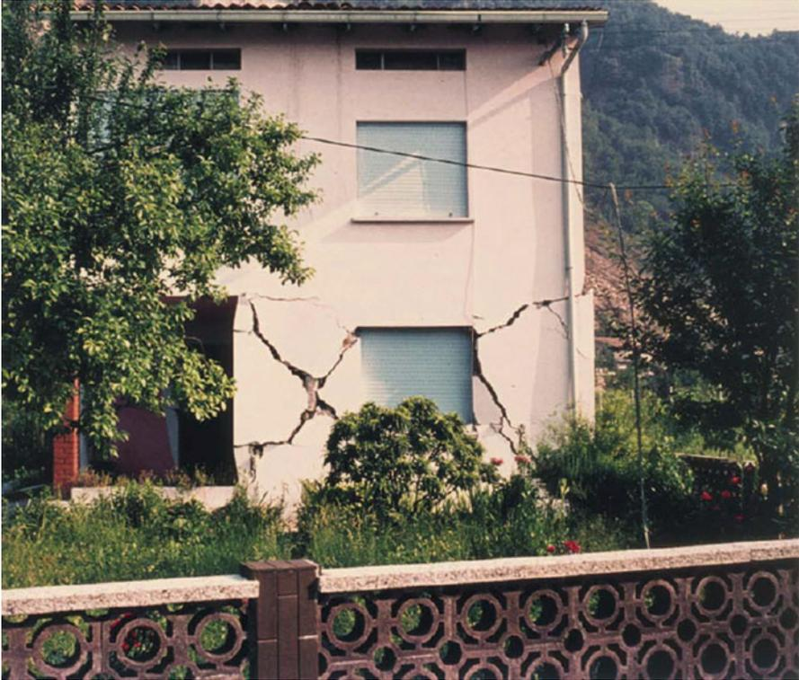
**Fig. 16.7** Unreinforced masonry with RC floors, grade of damage 4 (Grünthal 1998, EMS-98 scale)
