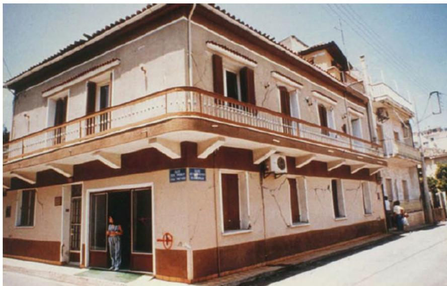
**Fig. 16.8** Unreinforced masonry with RC floors, grade of damage 3, in Greece 1995 (Grünthal 1998, EMS-98 scale)
